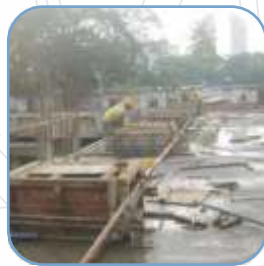
CIVIL WORK ON SITE
